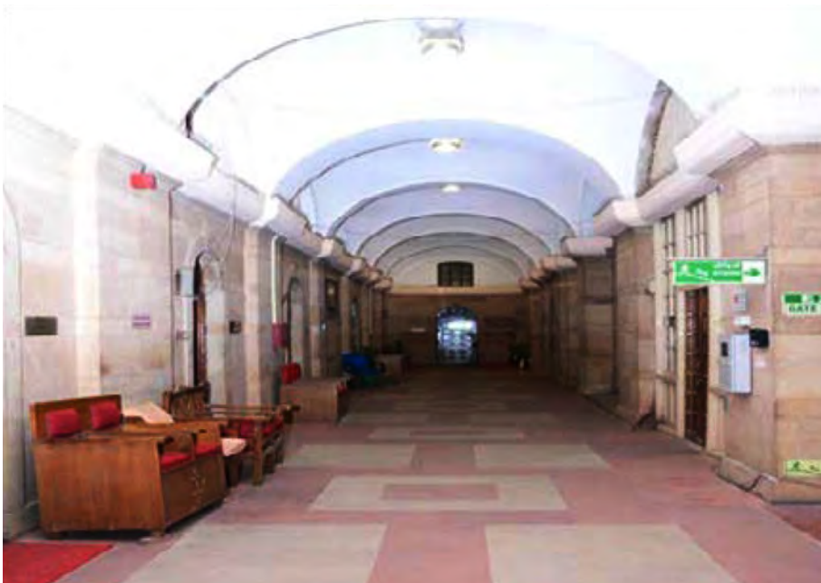
Replacement of stone on the walls and the corridors in the North and South Block, New Delhi; Source - Conservation and Audit of Heritage Buildings, CPWD
