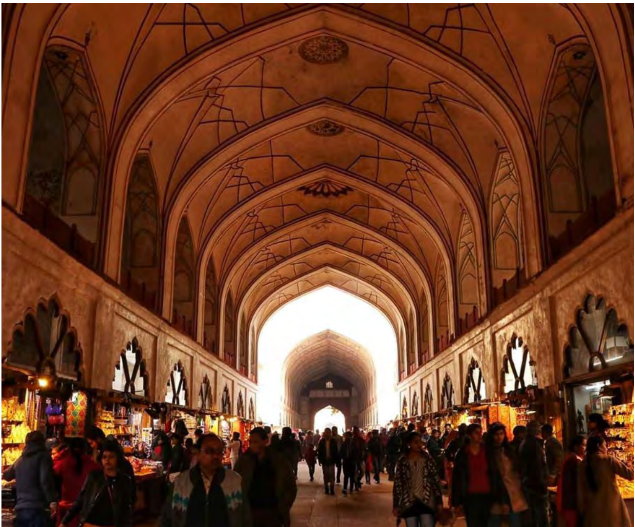
Before and after the restoration 2.4 Chatta Chowk, Red Fort of Chatta Chowk, Red Fort
