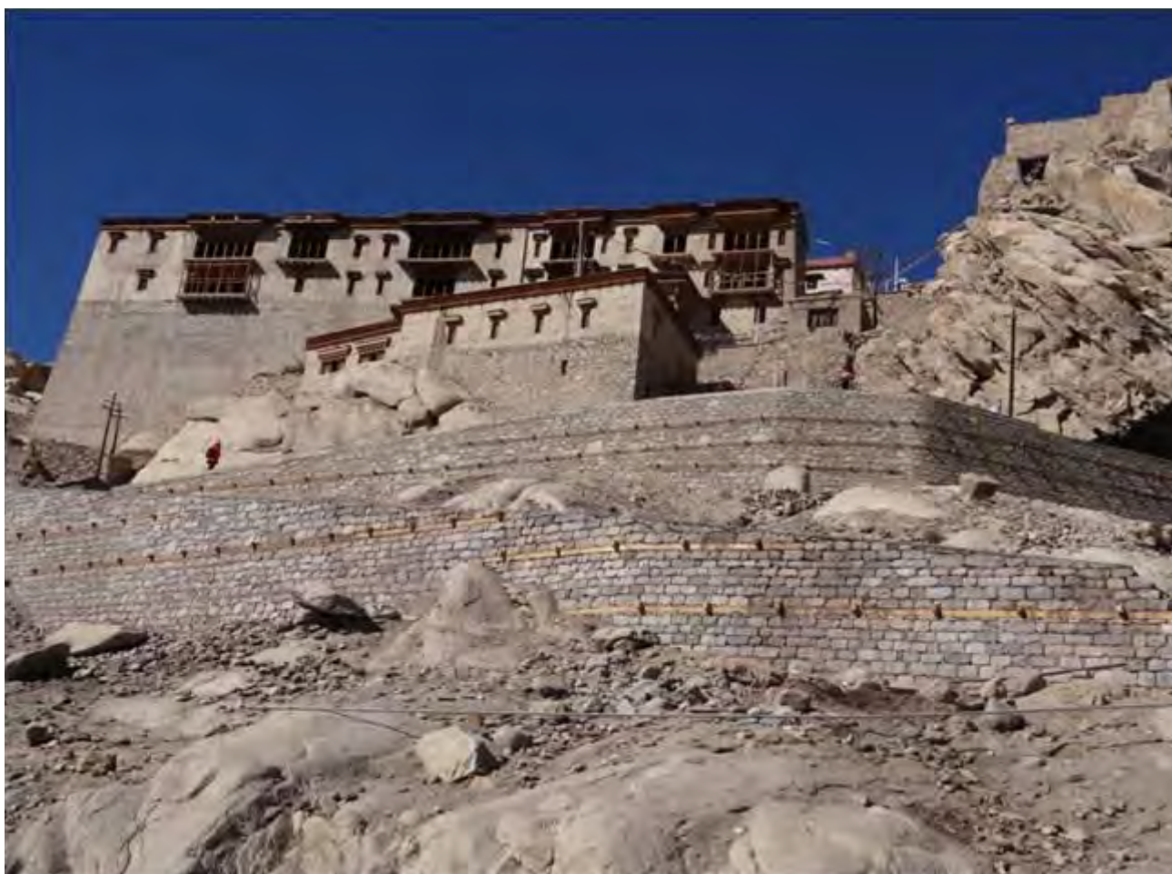
Before and after the structural conservation of Shey Palace
