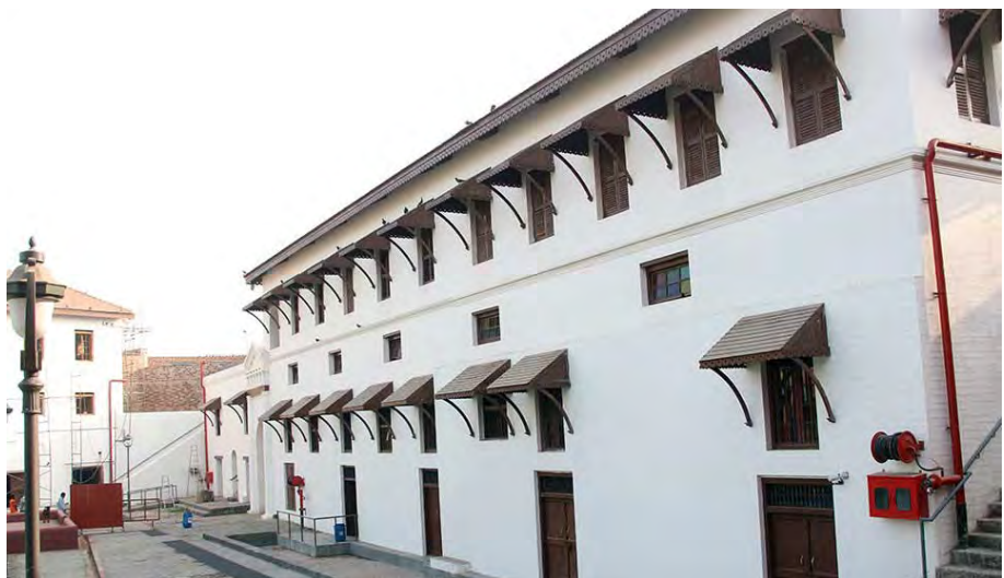
Restored Building housing the Mughal Gallery, Armenian Gallery, Trade Gallery, Court Room and Dutch Lifestyle Room in the Surat Castle; Source - suratmunicipal.gov.in/
