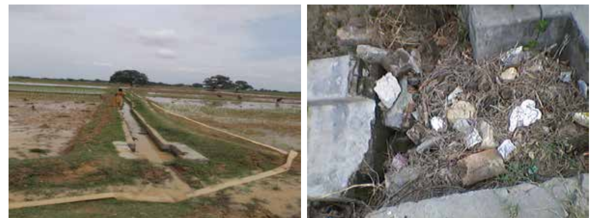
Photos of CADWM Works
